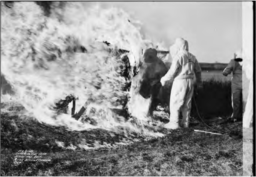
Demonstration of a Mansfield asbestos firefighting suit at R.C.A.F. Station Ottawa, 1939 Rockcliffe, Ont. (Library and Archives Canada)
