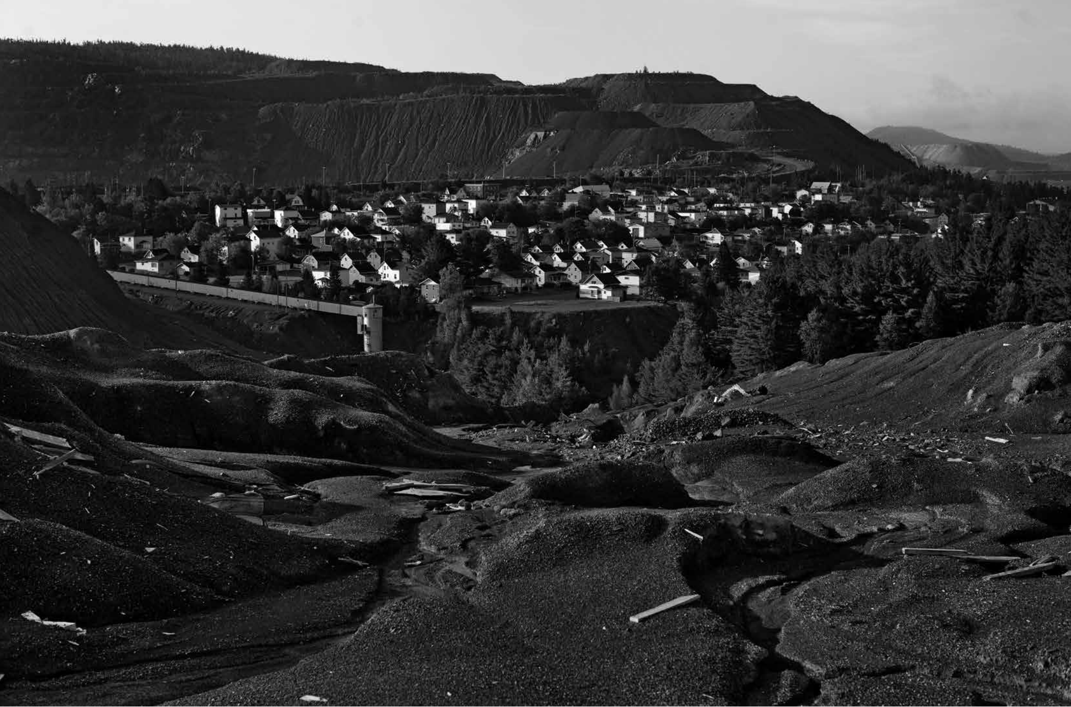
The town of Black Lake, Quebec, now a part of Thetford Mines, is surrounded by tailings and residue from the mining of chrysotile asbestos. Up to 300 million tons of this residue has been abandoned by mining operations throughout the region.
