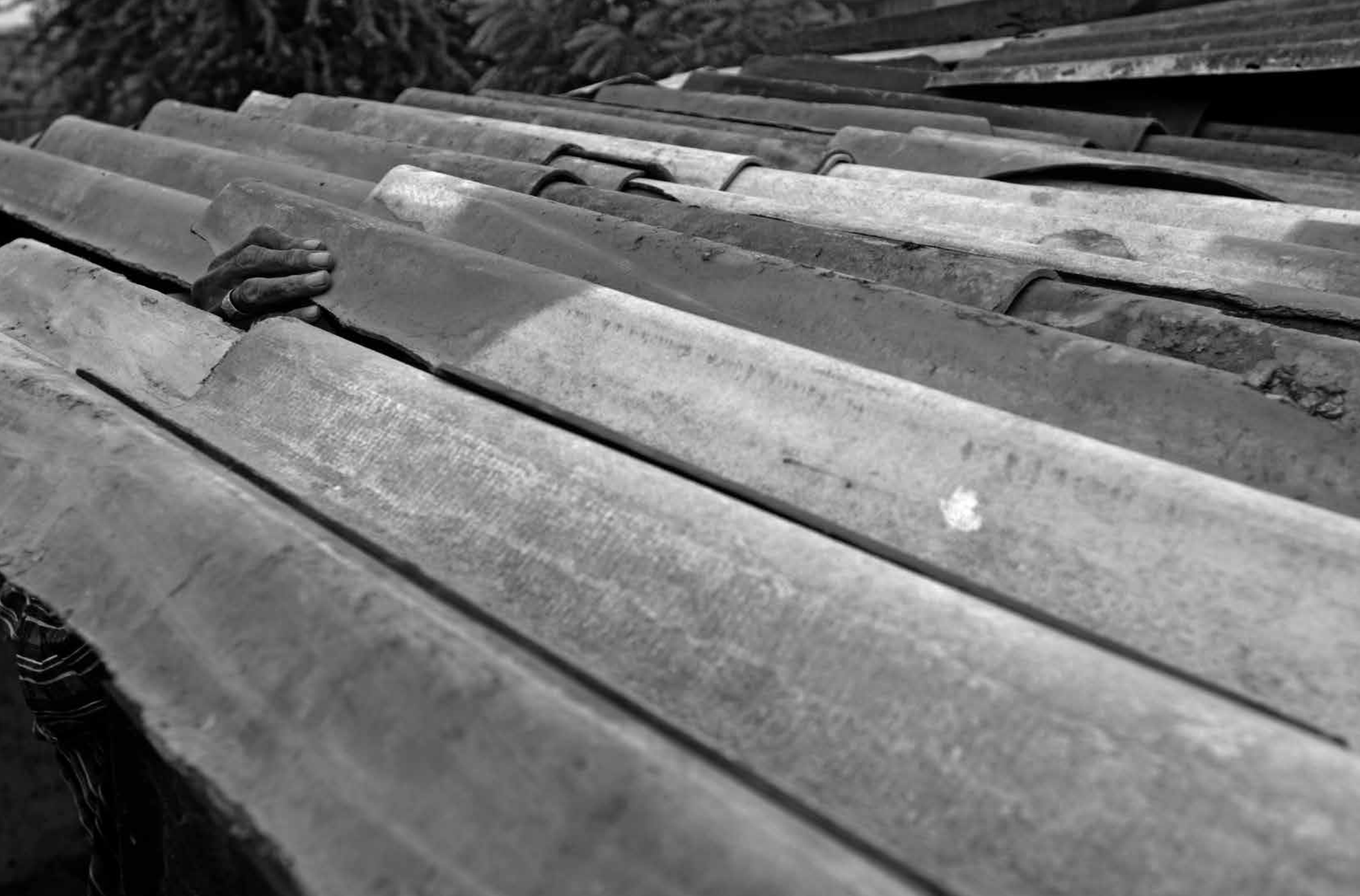
A man adjusts asbestos cement roof tiles on a house in a poor rural community on the outskirts of Ahmedabad, India. This entire community is built on top of—and from—the asbestos scraps from decades of production at a nearby cement plant. This man broke numerous pieces of roof tile containing asbestos wearing no protection.
